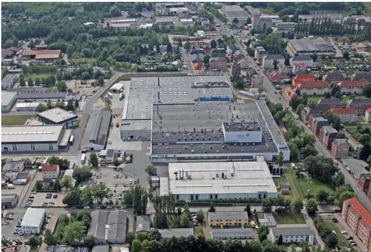
Aerial shot of the Johnson Controls battery plant in Zwickau, Reichenbacher Strafle. Photo: Johnson Controls, Ralph Koehler/propicture
